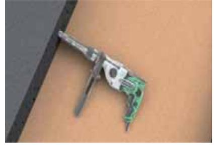
**Then drill and fix deformed bars ( $\phi 16 \times 600$  lg) in each concrete slab.
