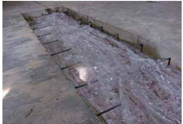
**Install a HC Sinus Slide® joint in the middle of the gap opening between the concrete slabs. Level out the HC Sinus Side® joints down and across. Eventually, weld the dowels fixed in the concrete slabs to the anchorage system of the HC Sinus Slide joint or use reinforcing mesh to link dowels and joint connectors.**
